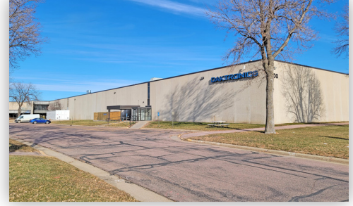
Daktronics Building 600 E. 54th Street N Sioux Falls, SD 238,875 sq. ft.
