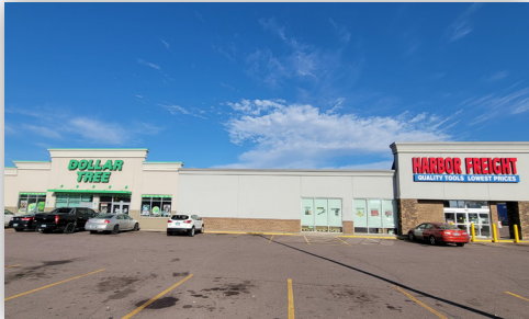
Harbor Freight Building 3100 W. 12th Street Sioux Falls, SD 34,678 sq. ft.
