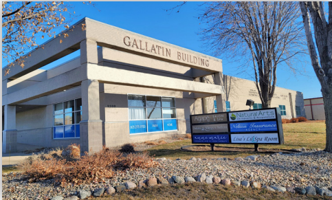
Gallatin Building 2200 W. 49th Street Sioux Falls, SD 14,873 sq. ft.
