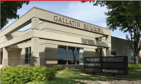
Gallatin Building 2200 W. 49th Street Sioux Falls, SD 15,000 sq. ft.
